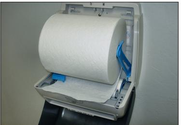
4) Install a new roll with the web coming off the back. Place tail of paper under transfer bar.
